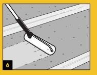
Apply one coat of Ready Roof liquid rubber at a minimum 1.6kg/ m2 using a roller on the deck or brush intricate or detailed sections. Leave overnight to cure before trafficking/walking on the finished surface.
